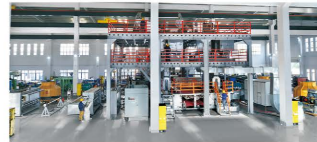
Double beams (SS)PP spunbond nonwoven fabric production line
